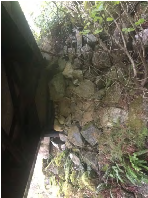
Left Bank Abutment when facing downstream
